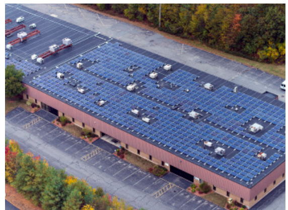
Parsons Commercial Group | 45 South St., Hopkinton 175 kW
